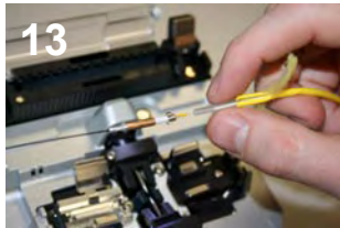
13 Slide 20mm protection sleeve over splice point, shrink in heat shrink oven.
